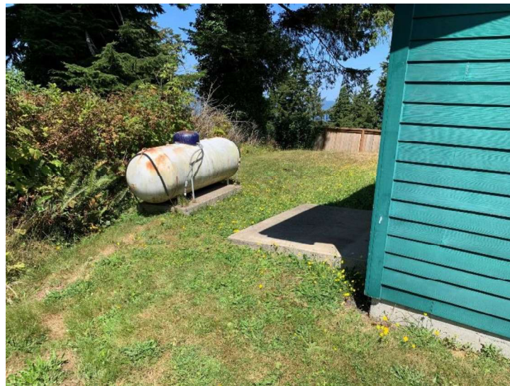
Figure 3.49 – Emergency Generator Propane Tank Near Top Edge of Slope
