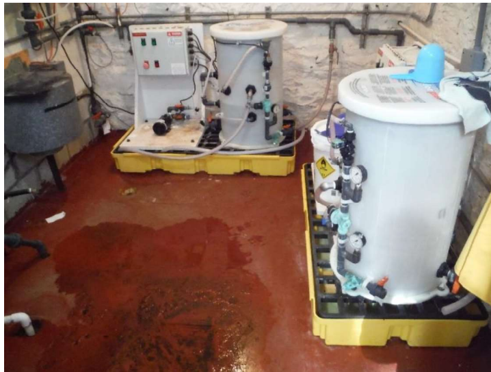
Figure 3.16 – Chlorination System and Spill Containment Skids not Adequately Restrained
