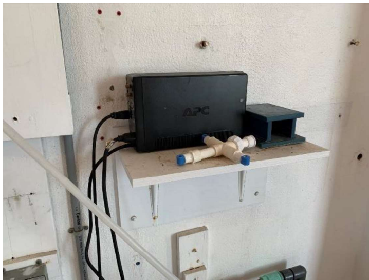
Figure 3.32 – Chlorination System Backup Battery not Adequately Restrained
