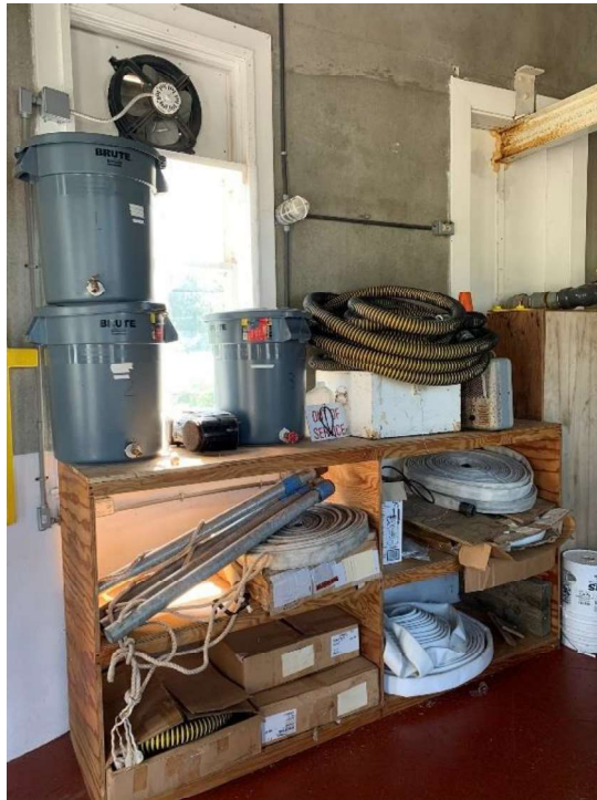
Figure 3.33 – Unanchored Storage Rack and Unrestrained Contents
