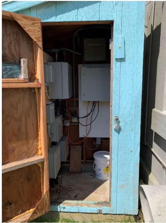
Figure 3.37 – Wood-Framed SCADA Enclosure with Limited Capacity to Resist Seismic Forces
