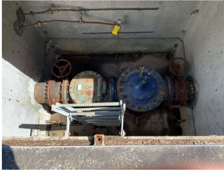
Figure 3.45 – No Flexibility at Pipe to Wall Interfaces and Valves Inside Altitude Valve Vault are not Independently Braced
