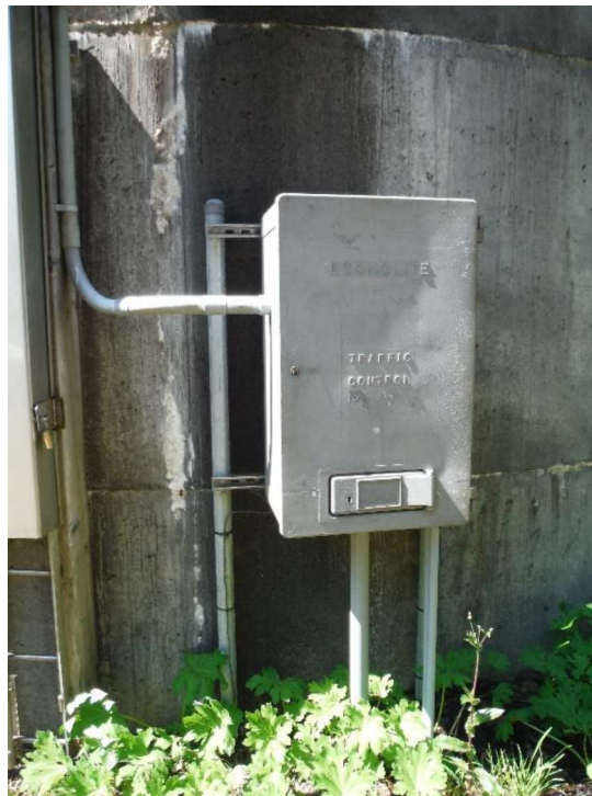
Figure 3.43 – Conduits from Below Grade Connecting to Chlorine Analyzer Cabinet without Flexibility
