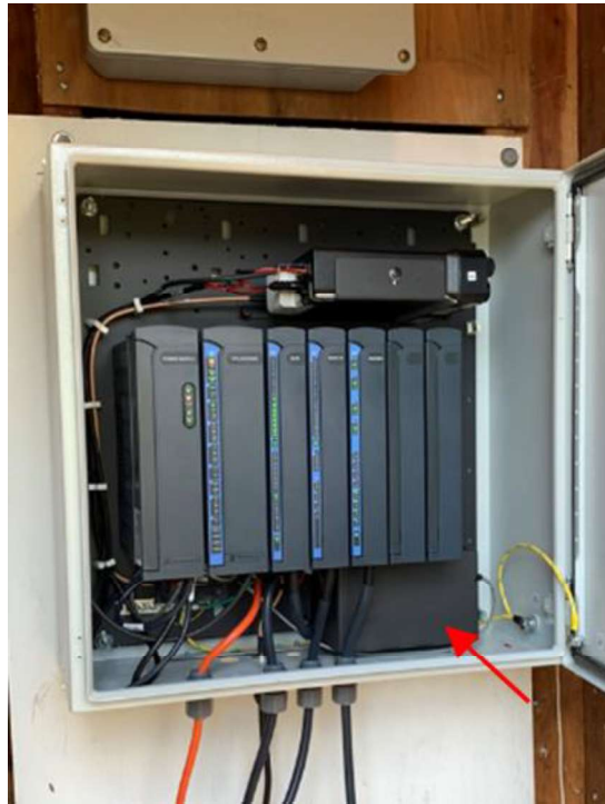
Figure 3.38 – SCADA Backup Battery not Adequately Restrained
