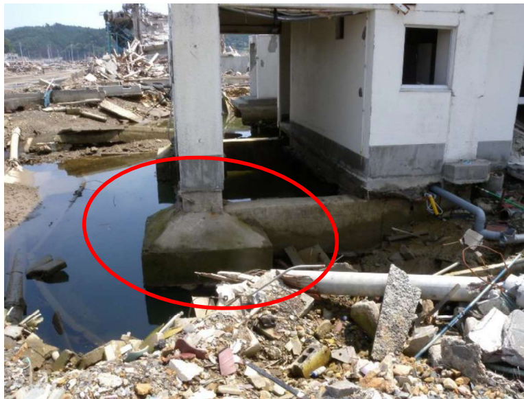
(a) Foundation and Pipelines Exposed Adjacent to Building
