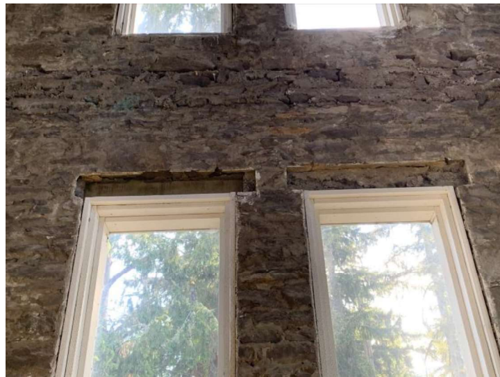
Figure 3.5 – Missing Partial Thickness of Wood Lintel Beams Above Window Openings
