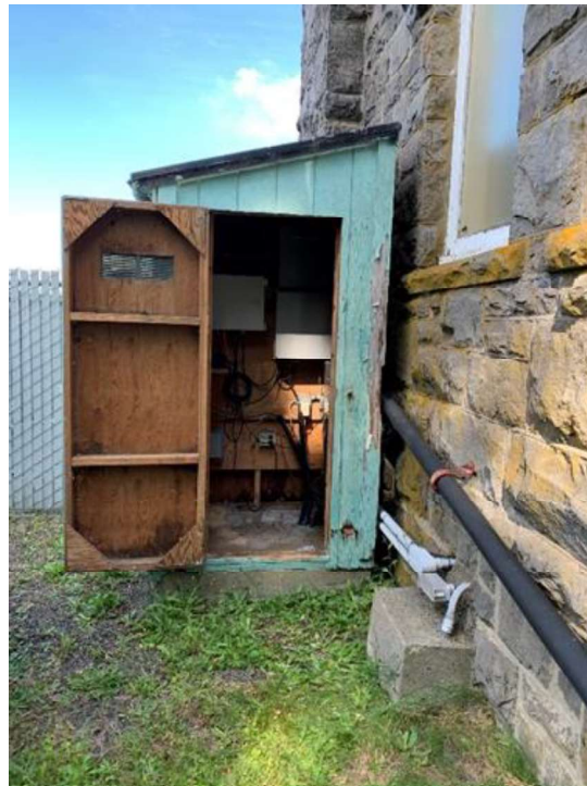
Figure 3.20 – Wood-Framed SCADA Enclosure with Limited Capacity to Resist Seismic Forces
