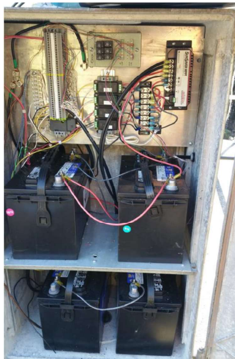
(b) SCADA Batteries not Adequately Restrained
