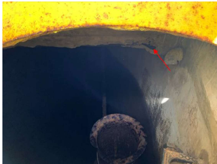
(b) Composite Floor Beam in Gate Well
