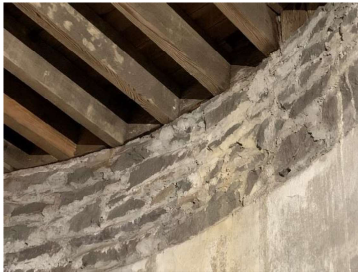
(b) Joist-to-Wall
