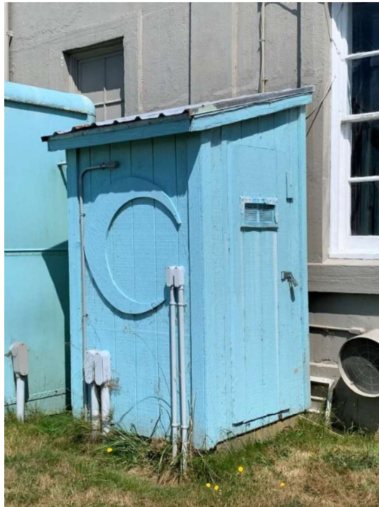
Figure 3.26 – Reservoir 3 Wood-Framed SCADA Enclosure
