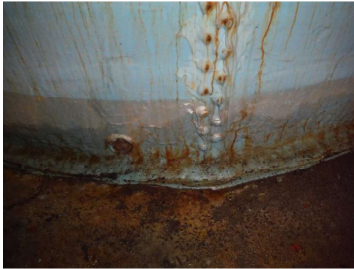
Figure 3.15 – Steel Tank Lacks Anchorage to Resist Sliding and Overturning
